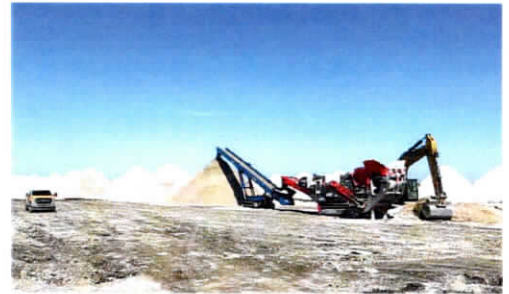
Construction continues on the STA Inflow/Outflow and Seepage Canals.
