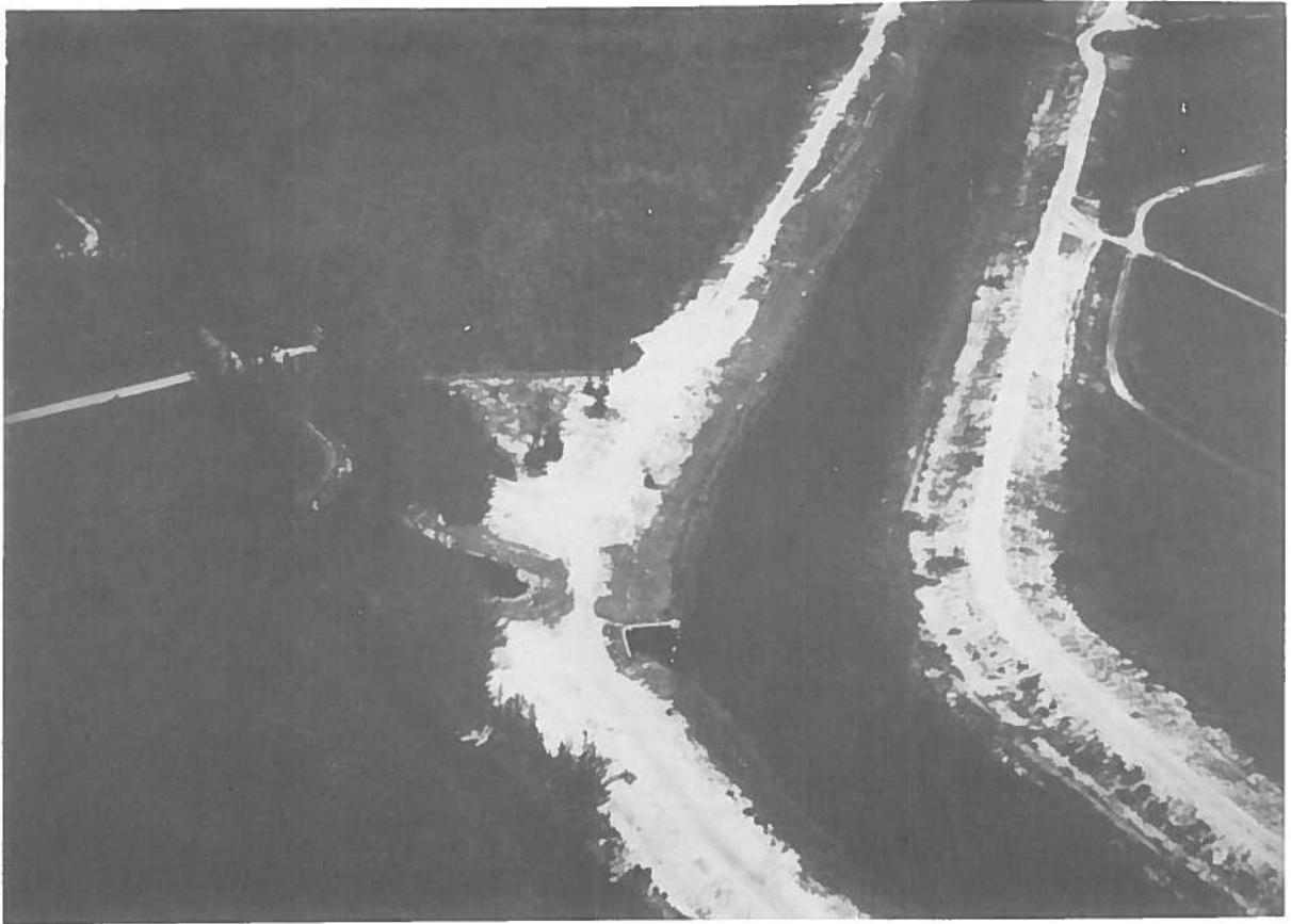
River Mile 14.5 - The Loxahatchee River (left) Flow is Augmented by the C-18 Canal System (right) Culvert Diversion
