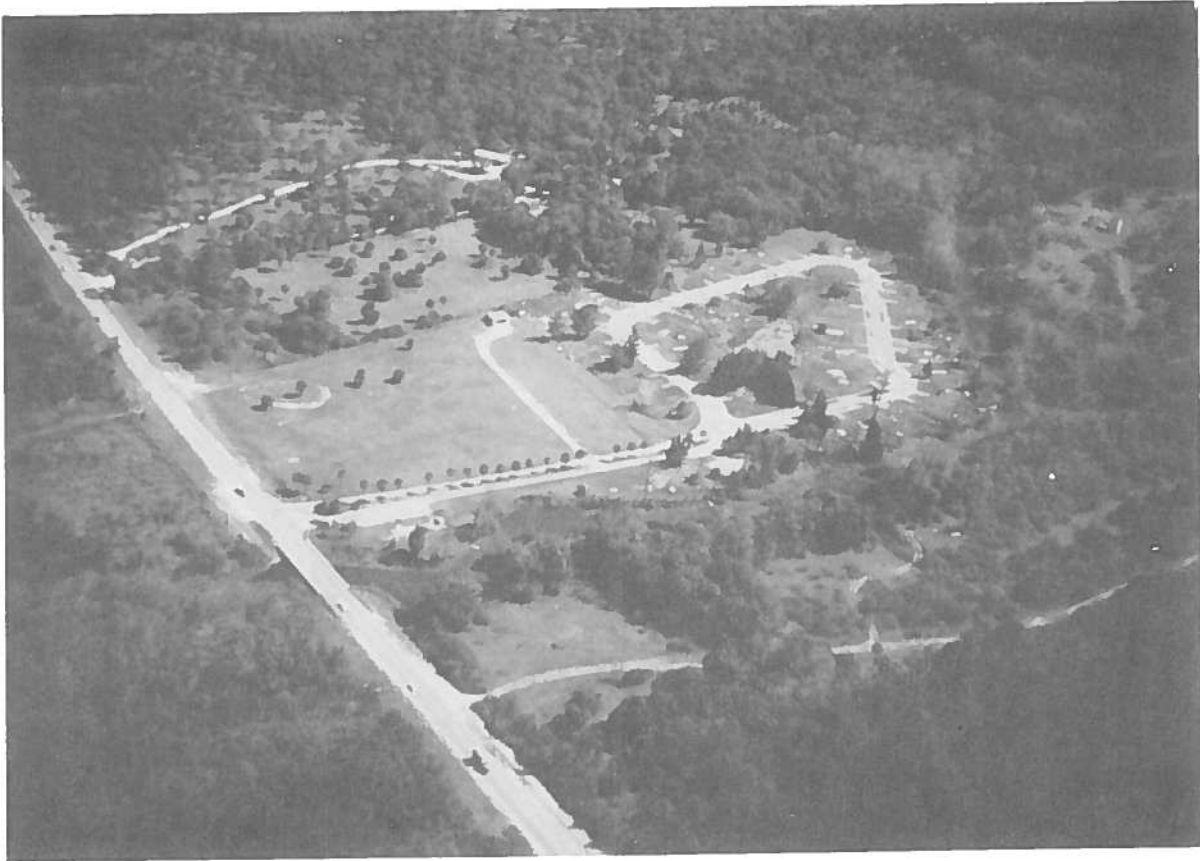
River Mile 13.5 - Palm Beach County has Purchased a 187-Acre Site Along the Loxahatchee River at Indiantown Road. The County Removed an Existing Trailer Park and Plans to Develop the Site as a Passive Recreation Park Focused on the River
