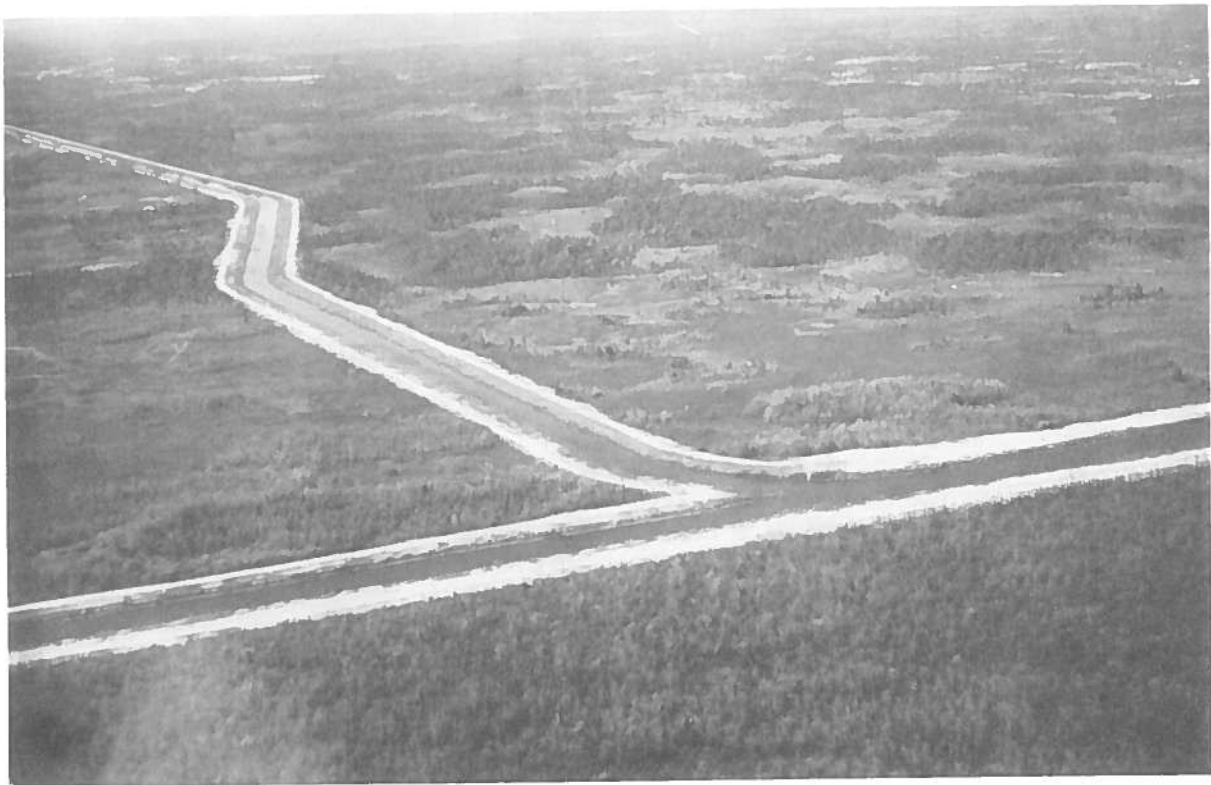
The C-18 Canal System Drains the Loxahatchee Slough
